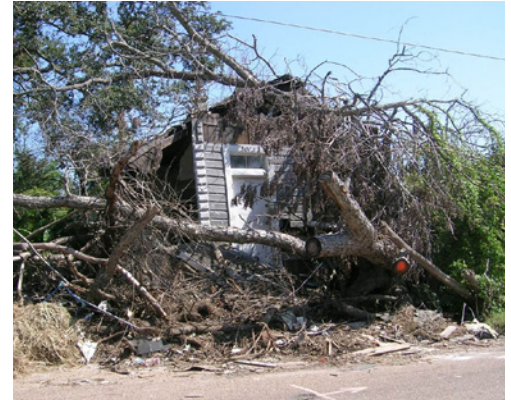
Photo 1: Hurricane Damage in the Ninth Ward, New Orleans
