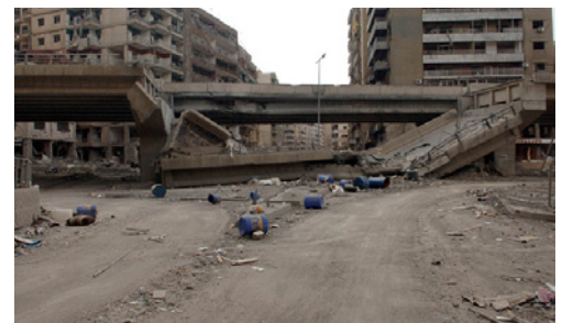
Photo 2: Damage from the 2006 War in Lebanon
